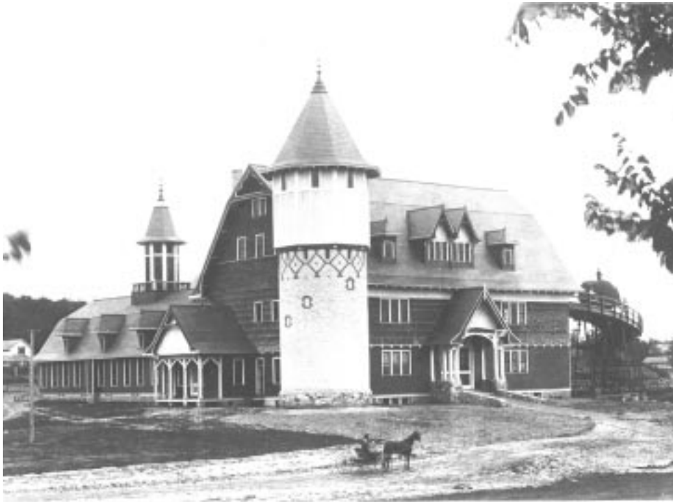
Fig. 2. The Dairy Barn about 1905 showing spiral ramp in rear (west) of barn. A team of horses pulling a loaded wagon could enter the third level hay loft directly by climbing this ramp. [x25-336]
