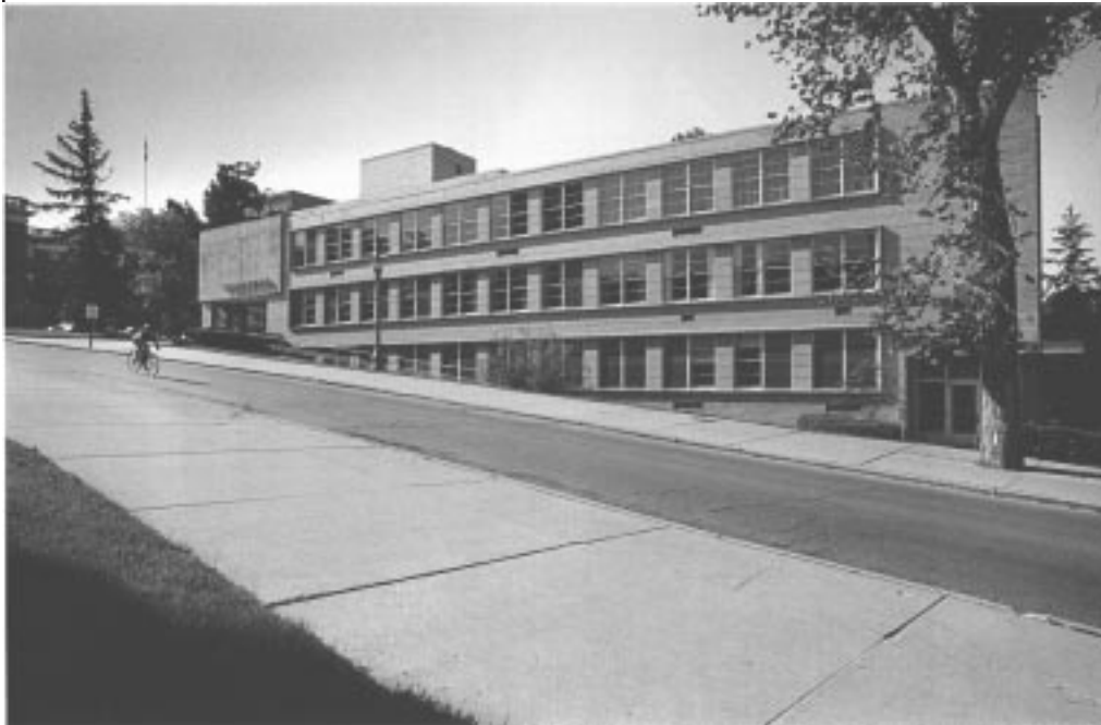
Fig. 1. The Commerce building, from the corner of Charter and Observatory Drive, 1959. The first of the "modern" buildings on the upper campus, the strong horizontal lines, are broken by the vertical stone panels, and still do not quite abandon the illusion that the outer walls are load bearing. [Series 9/1, Commerce, jf-70]
