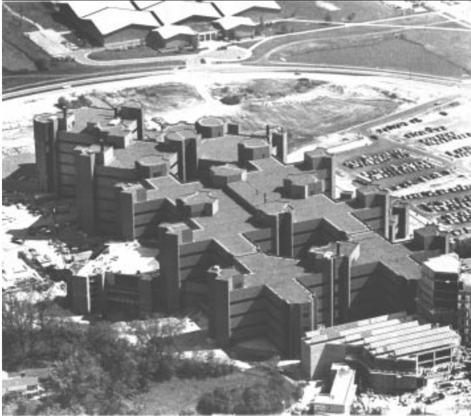
Fig. 1. The "completed" Clinical Science Center. Clear visible is the modular nature of the building, with the towers being stacks of modules connected at their corners. Nearly indefinite expandability is a hallmark of the design. The building in the background is the Nielson Tennis Stadium. [7/4 folder #2, jf-97]
