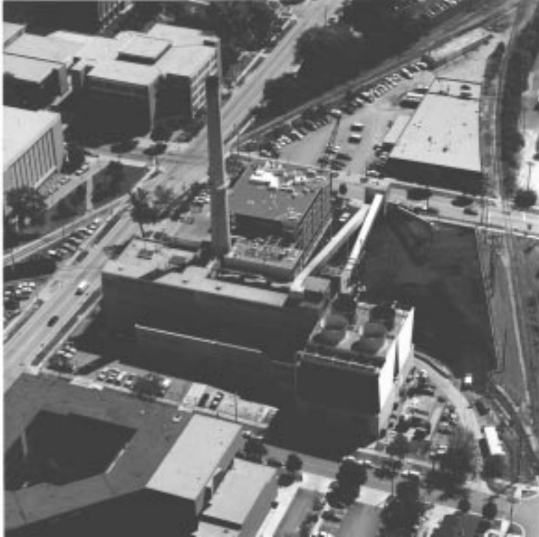
Fig. 1. The Charter St. Heating plant looking east c. 1985. The emission control "bag house" is under construction on the east side of the plant. Dayton Street is at the left of the picture. The single smokestack was built in 1963 to replace the original three shorter stacks, which were too low to prevent soot in the neighborhood. [series 9/5, Charter Street Plant, jf-74]
