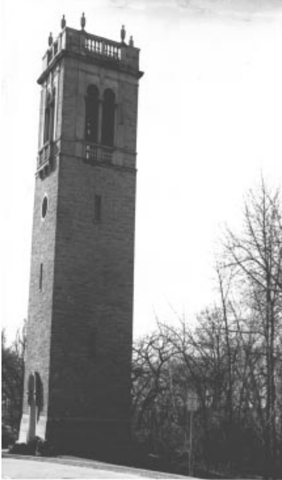
Fig. 1. The carillon tower c. 1938. [Series 9/1, Carillon, jf-57]
