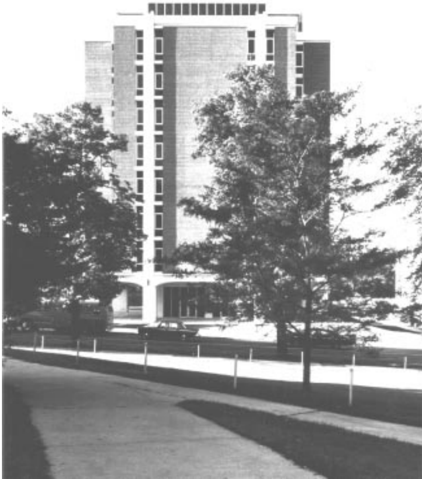
Fig. 1. Bock Labs from Linden Drive c. 1968. Forty feet from Agricultural Engineering on the east, and 55 feet from Moore Hall on the west, Bock Labs is connected by tunnel to the Biochemistry building to the south. Bock Labs has two levels below ground and seven stories above ground. [Series 9/3, Biophysics - Molecular Biology, jf-84]
