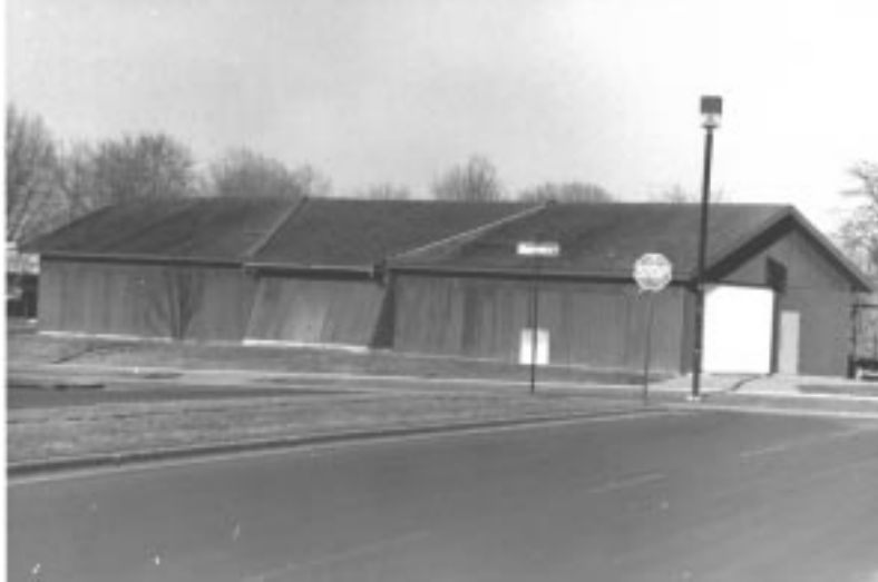
Fig. 1. The Band Storage building, 1995. The building is one story 36 by 100 feet of reinforced concrete with plywood siding and cedar shingles. It was designed to require minimum maintenance, and has an estimated 50 year lifespan. [Author Photo, AP-60]
