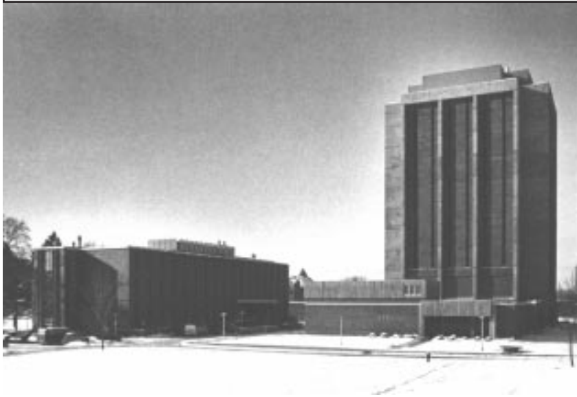
Fig. 1. The animal science building at the right, veterinary science at the left, 1975. The electron microscope is housed in the low section in the foreground. [series 9/3, Animal Science, jf-93]
