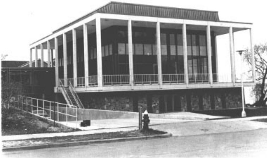
Fig. 1. Alumni House from Lake Street c. 1967. It is a three story building of steel and reinforced concrete, with Wisconsin field-stone sheathing on the lowest level. At left is the connecting link to the Wisconsin center. [series 9/2, Alumni House, jf-83]
