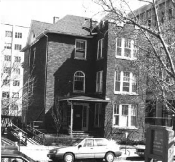
Fig. 1. Spring 1994: 433 N. Murray Street, built about 1910 as a replacement for an older family house, the third floor was added in 1914. The building was used as University offices, starting in 1966, and was demolished in 1994. [Author Photo AP-2]
